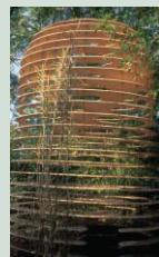
This spiral staircase is made from suspended sheets of timber cut to shape and spaced about six inches apart. Children can climb inside the structure, which is the focal point to Pascale and Christian Pottgiesser's garden 'The cat burglar'.
